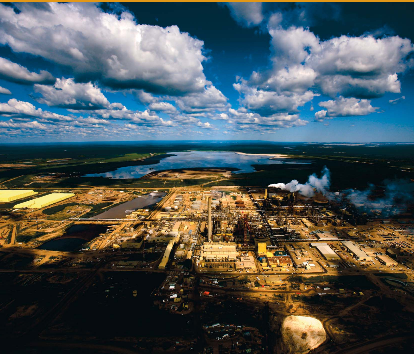
SYNCRUDE UPGRADER AND TAILINGS POND, ALBERTA, CANADA
