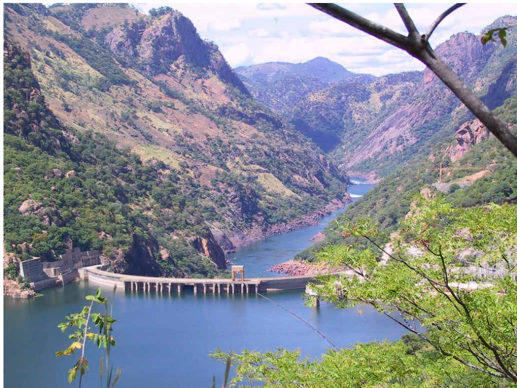
Cahora Bassa Dam in Mozambique. Credit: Ryan Hoover
