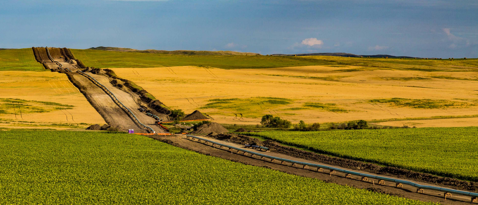
Construction of the Dakota Access Pipeline near New Salem, North Dakota. Tony Webster. (CC BY-NC-SA 2.0)
