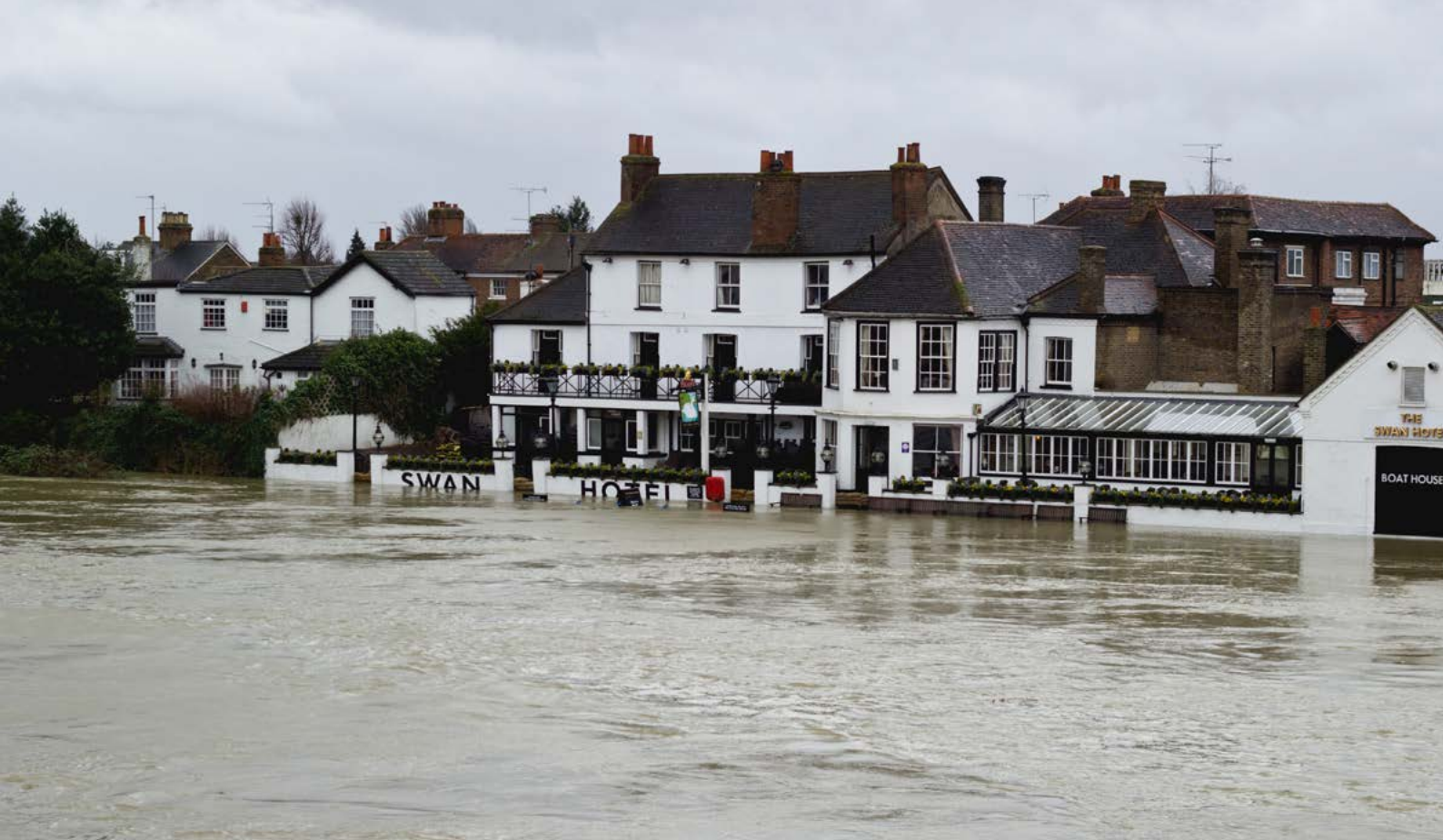
Flooding in Staines-upon-Thames during the historic 2014 UK flood event, which many studies have attributed in part to climate change. ©Marcin Cajzer (CC BY 3.0)
