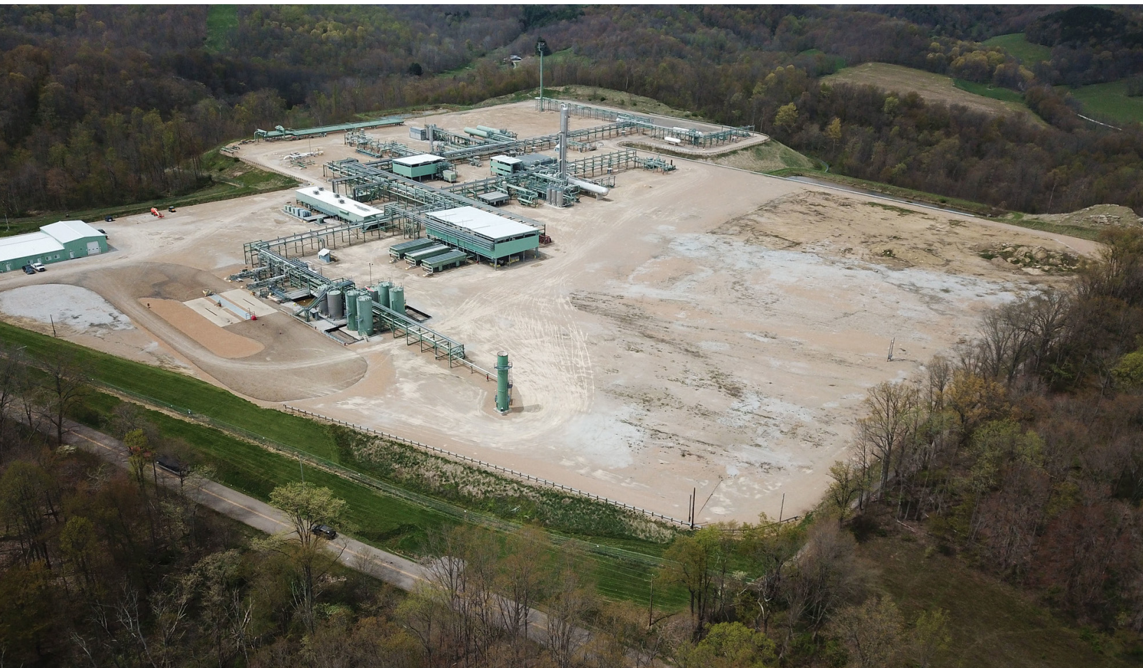
A gas processing plant in Carroll County, Ohio. ©Ted Auch, FracTracker Alliance, 2021.
