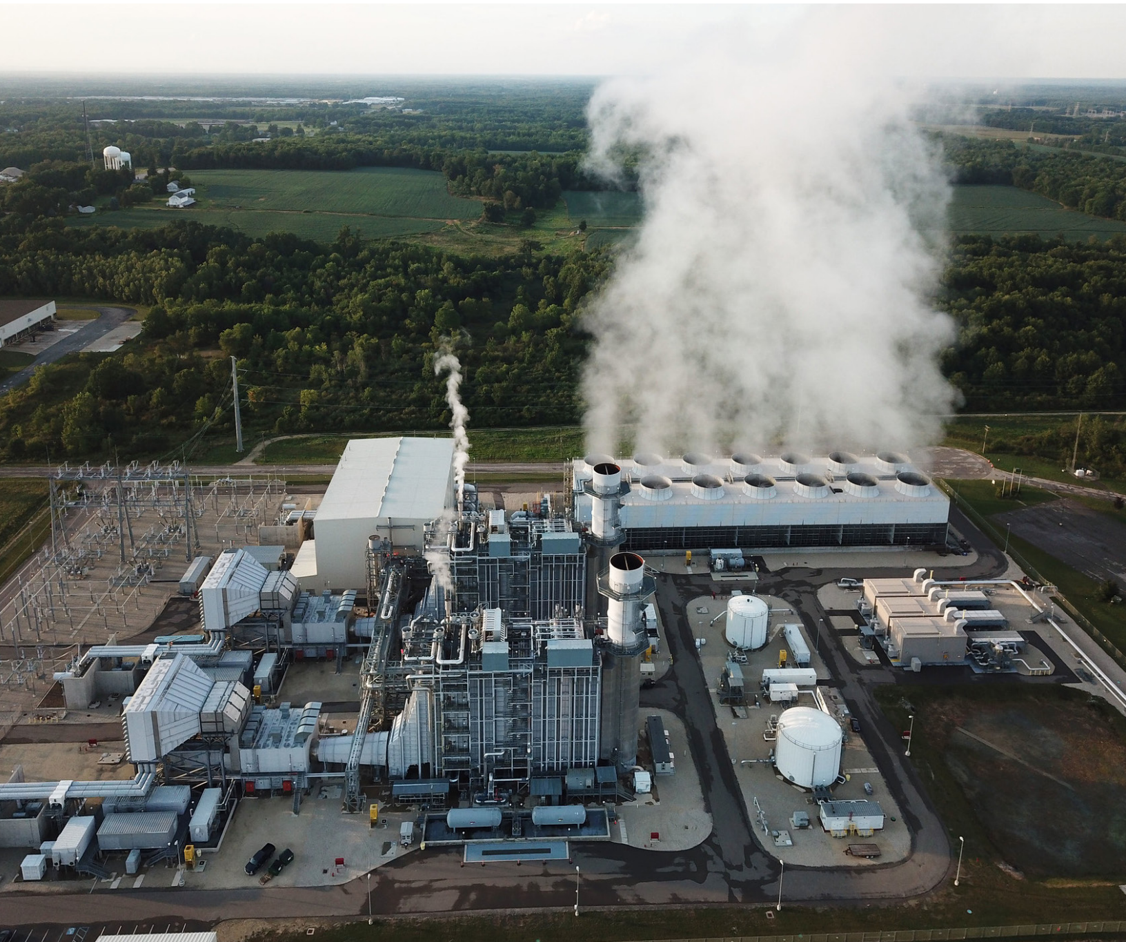
A gas power plant in Trumbull County, Ohio.. ©Ted Auch, FracTracker Alliance, 2021. Aerial support provided by LightHawk.
