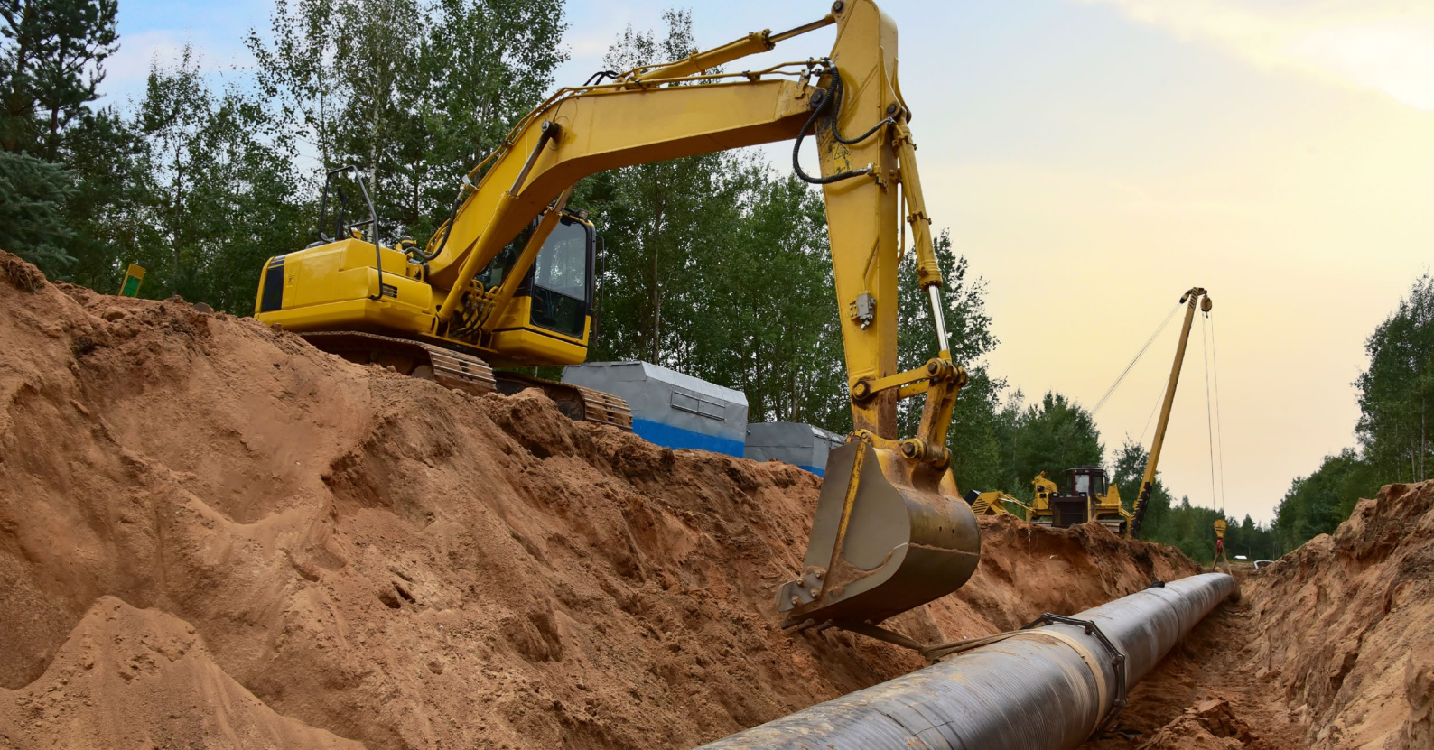
Gas Pipeline Construction, by MaxSafaniuk, Adobe Stock stock.adobe.com
